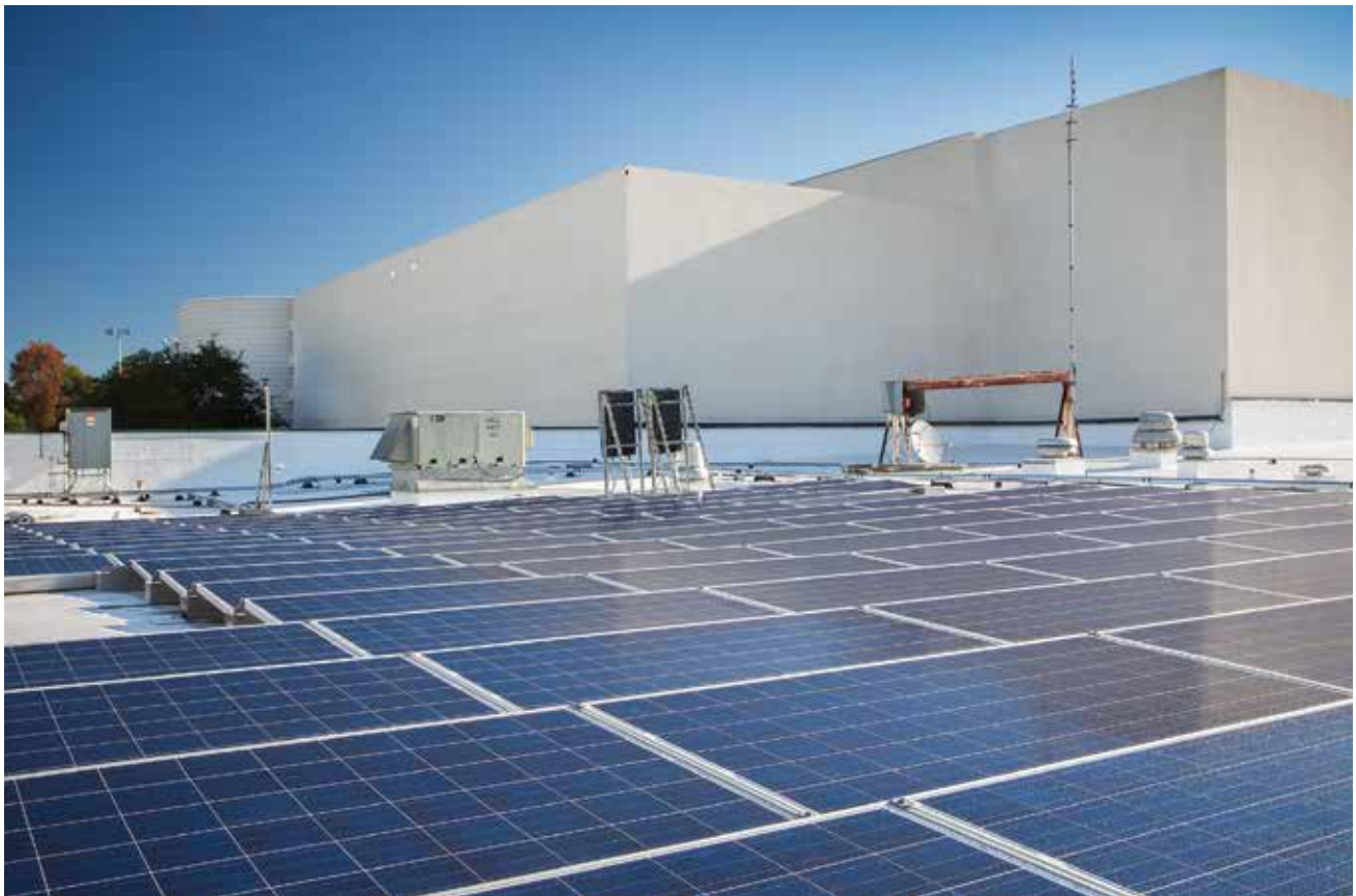
Columbiana Centre's 300 kW solar installation is one of the largest customer-owned solar generation facilities on SCE&G's system.
